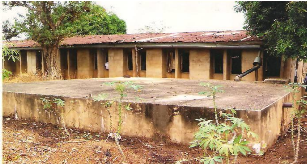
Plate 2. Rain Water From Tank In Effium: Front View
